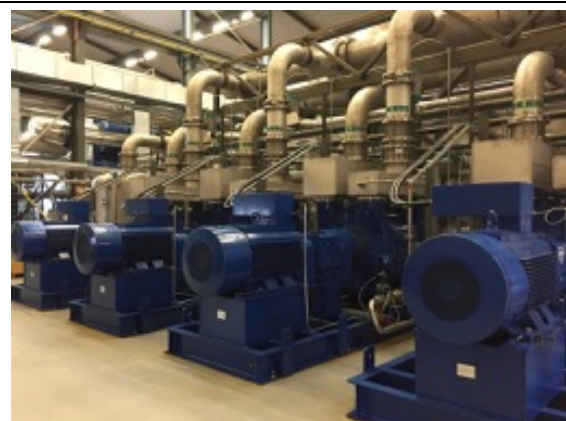
Photo 46: Gas vacuum pumps
