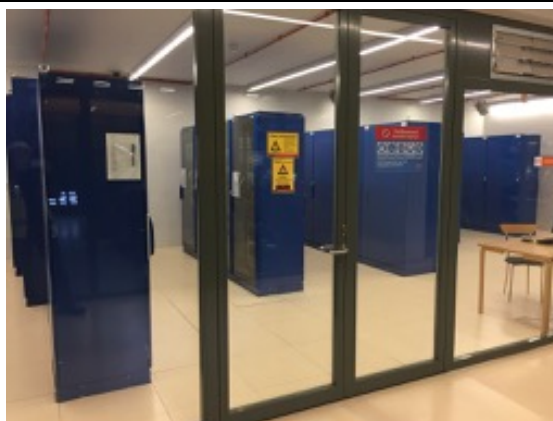
Photo 52: Electric controls in overpressurized room (protected from H 2 S)
