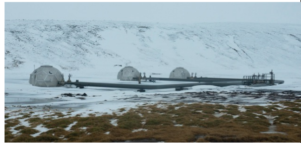
Photo 20: Reinjection wells
