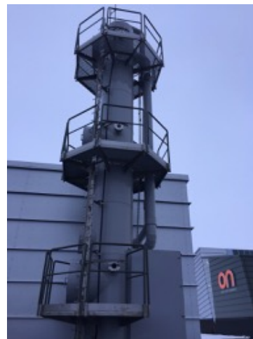
Photo 94: Scrubber for H 2 S and CO 2 reinjection
