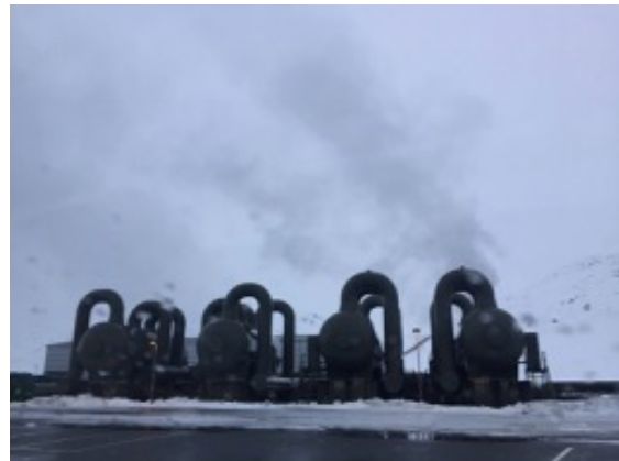
Photo 6: Demisters to produce dry steam
