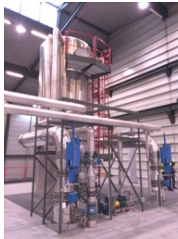
Photo 54: De-aerator in hot water plant
