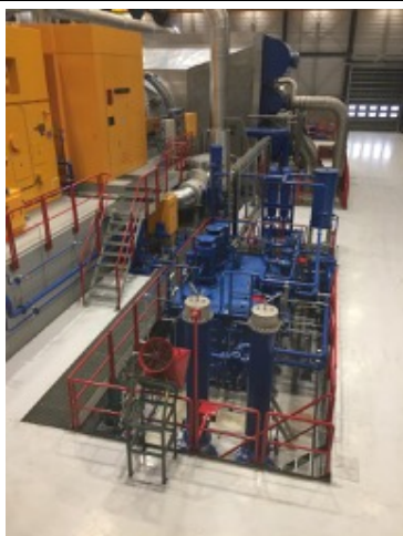
Photo 47: Sump next to generator, with oil pumps and fire control system
